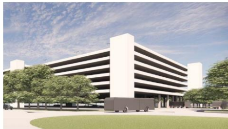
Figure 81. Airfield View of Car Park Y Multi-Storey Car Park and Flood Storage
